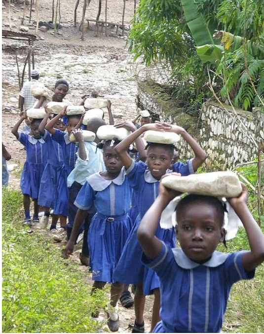
Students carry rocks from the dry riverbed to the school construction site, helping to build their own school buildings
